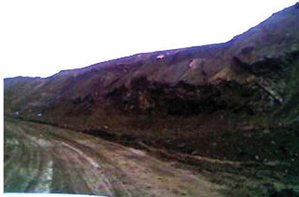
Fig. 3. Slope placed on the right hand of the road.
