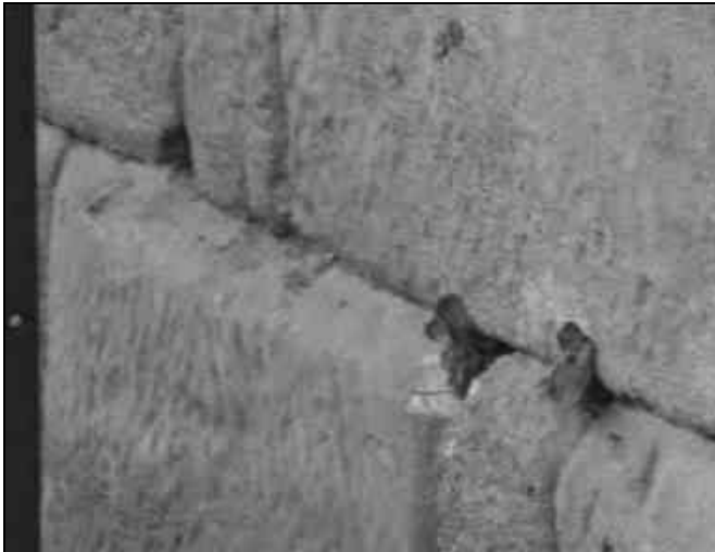
Figure 7. Exemplification of the chamfering technique used limestone blocks at Tilisca city
